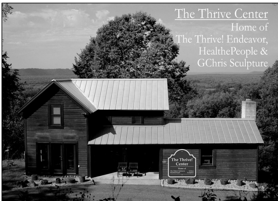
Thrive! Center Main Building, Renovated/Restored Farmhouse, 1885 Era
