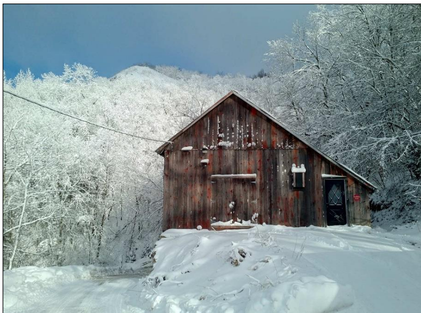
Thrive! Center Barn, Renovated/Restored, 1885 Era
